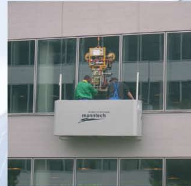
Auxiliary hoist to transport glass panels and elements outside the cradle (platform)
