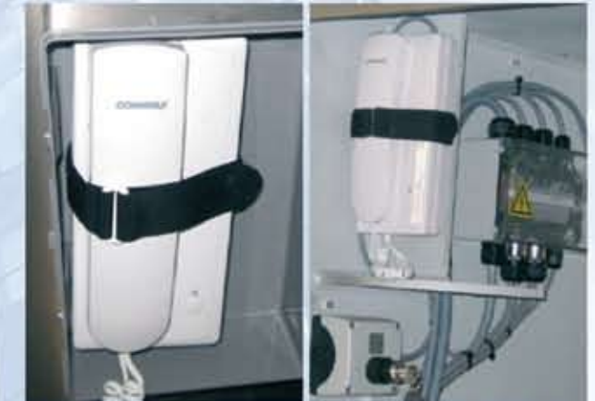
Telephone communication between cradle (platform) and roof car via control device in the ropes
