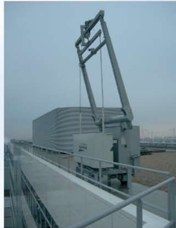
Rotating head for cradle (platform) guidance and consequent improvement of operating conditions
