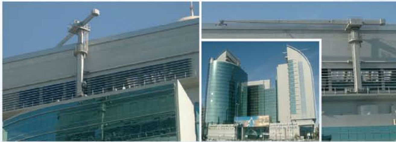
Type 6.2 with telescopic slewing mast and maintenance platform for hidden parking position
