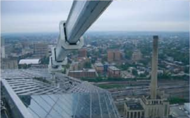
Type 6.1 with quadruple telescopic jib and vertical telescope mast, completely retractable on the roof
