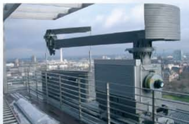
Slewing head with asymmetrical cradle attachment for circumnavigating obstacles
