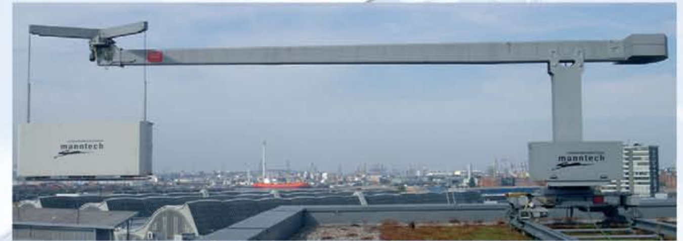
Type 6.1 with standard slewing head and fixed mast
