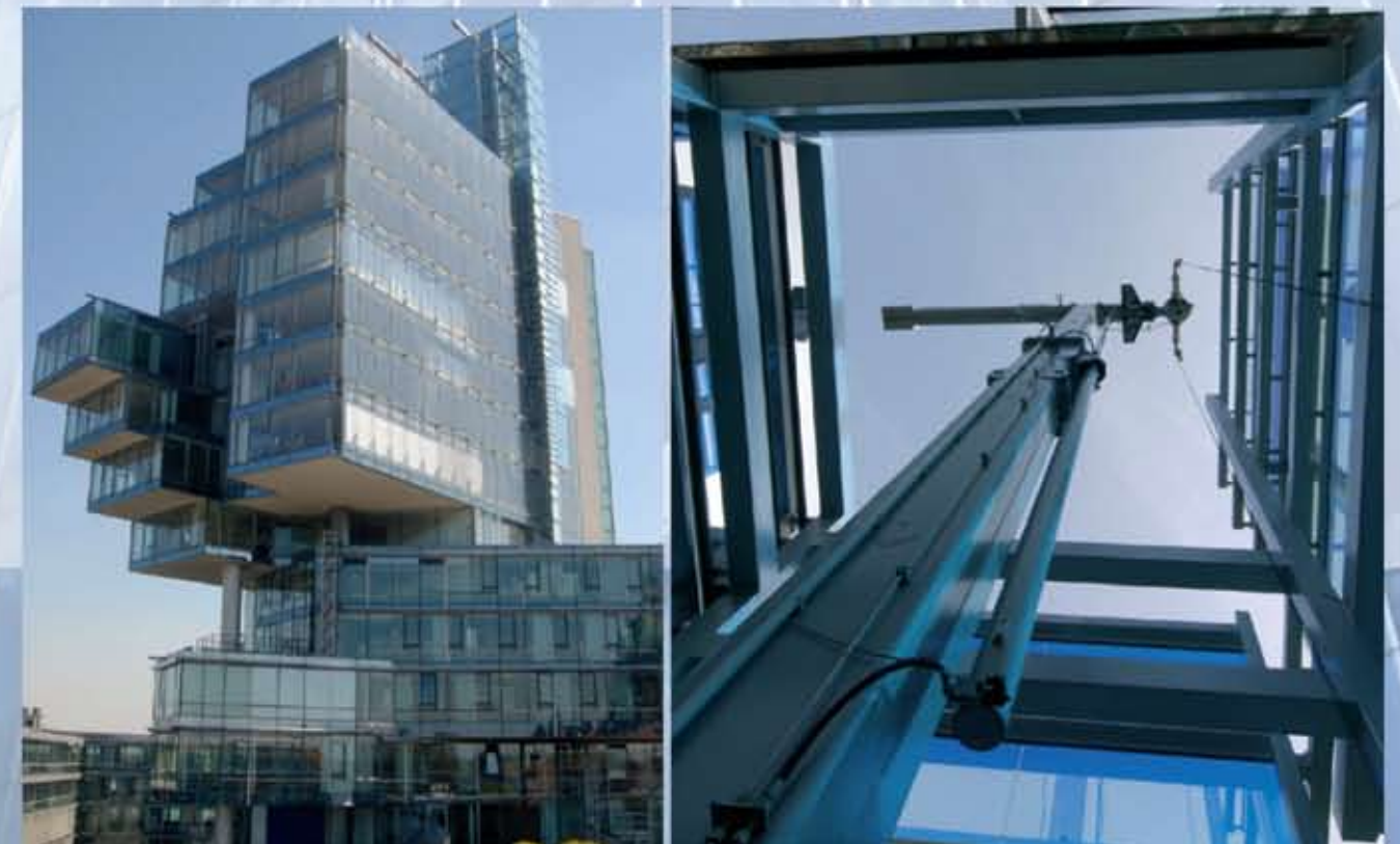
Type 6.4 with extremely high telescopic slewing mast
