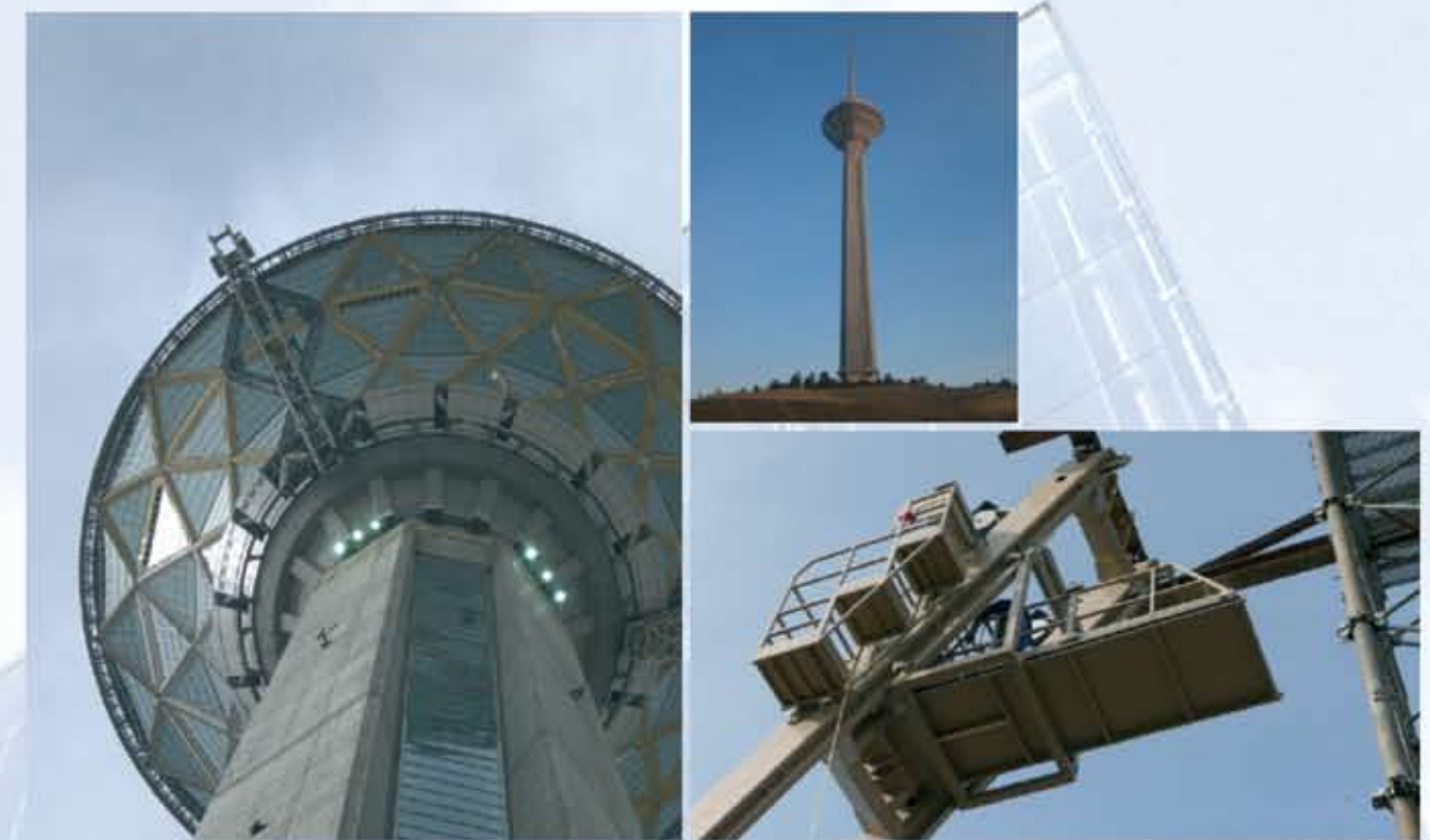
Milad Tower, Iran: Sloped elevator for maintenance of tower cupola. Designed for extreme wind stress and seismological conditions
