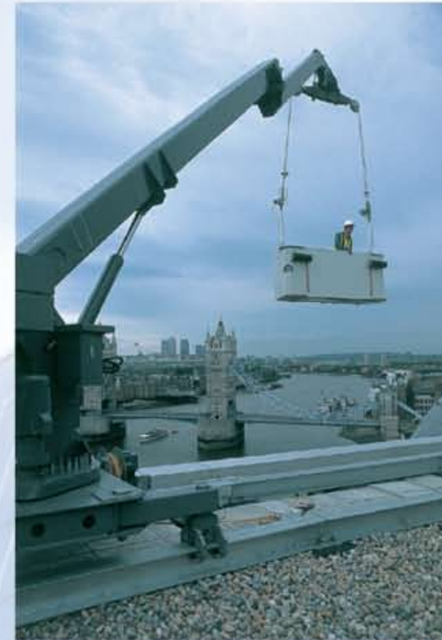
Type 6.1, track-based with fixed luffing jib and horizontal slewing articulation
