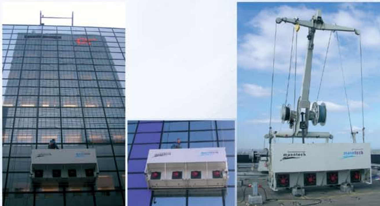
Delftse Poort, Rotterdam: Automatic cleaning machine
