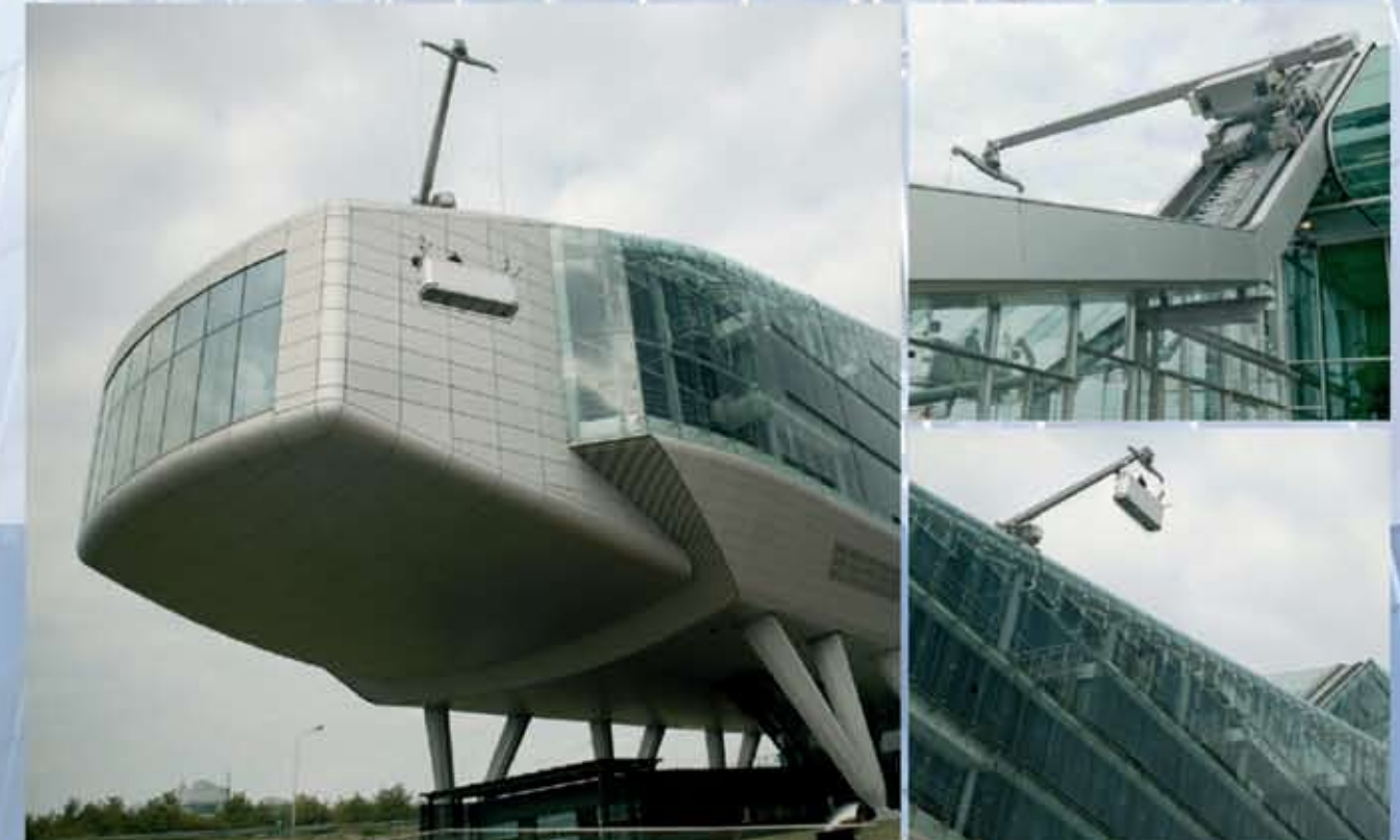
ING Bank, Amsterdam: Sloped track sections with a Type 6.1 machine, here with rack and pinion drive and slewing head in a special design
