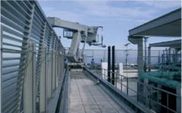
Type 6.1 with lowering device, triple telescopic jib and satellite cradle for reaching recesses in building
