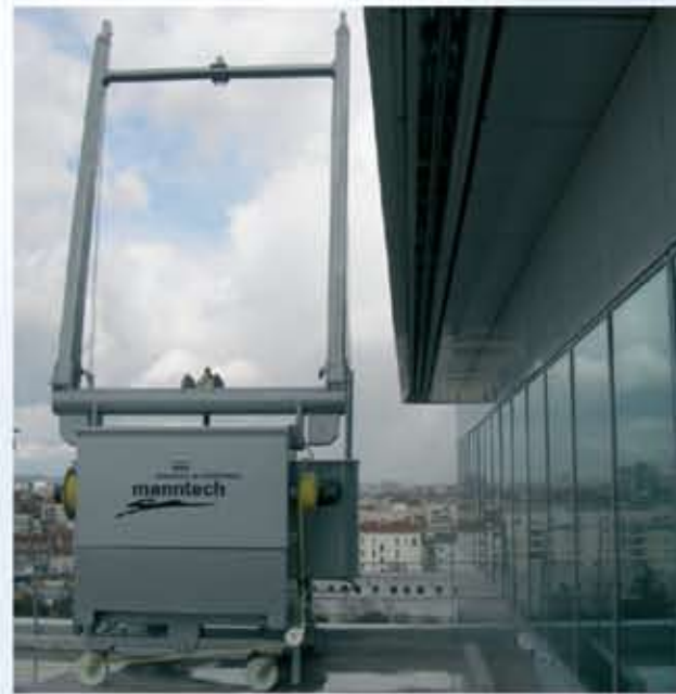
Type 1.3 with crossbar for load-bearing hoist
