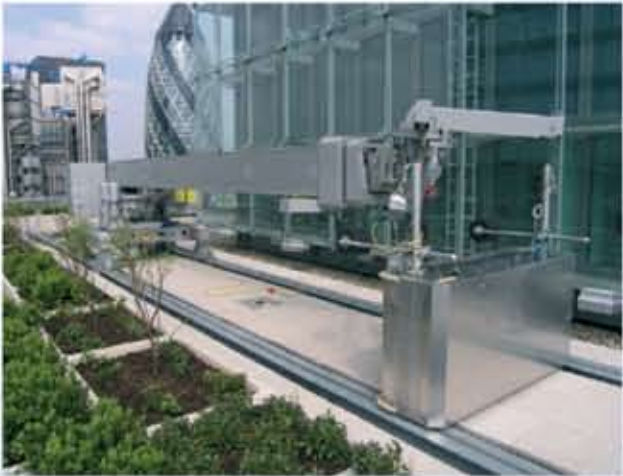
Type 6.1 in low profile construction with double telescopic jib, track system integrated in green roof system
