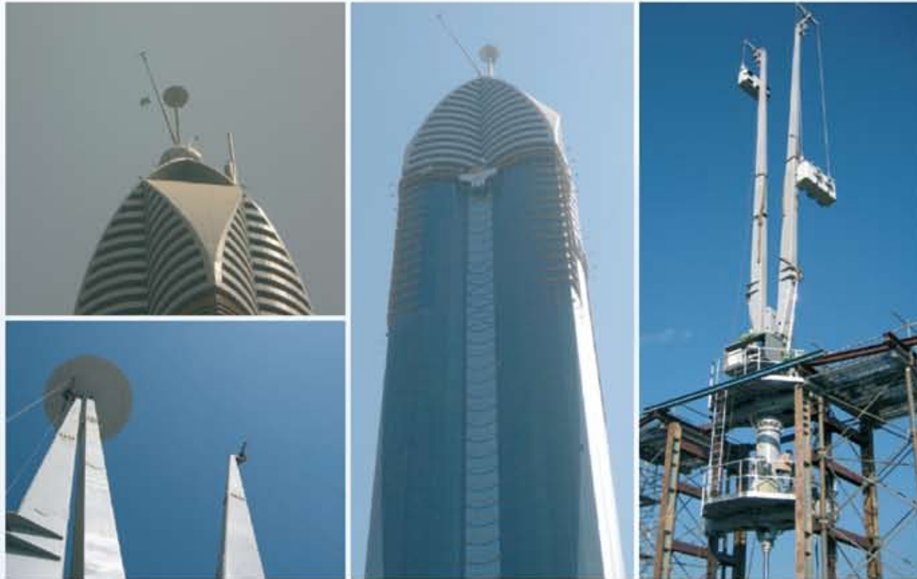
Rose Rotana Hotel, Dubai: In domed building, retractable crane type machine with twin jibs for optimal cleaning service
