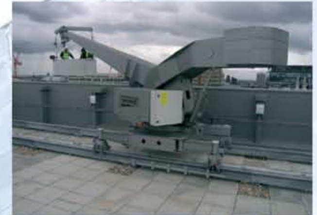
Type 6.1, track-based with fixed luffing jib, low-profile design
