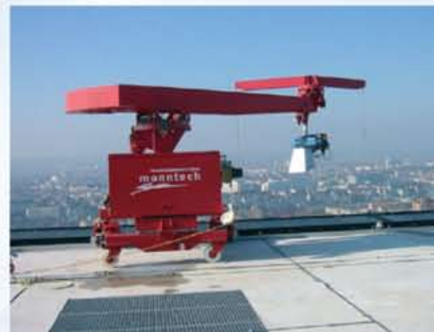
Type 4.3 with guide rail along parapet
