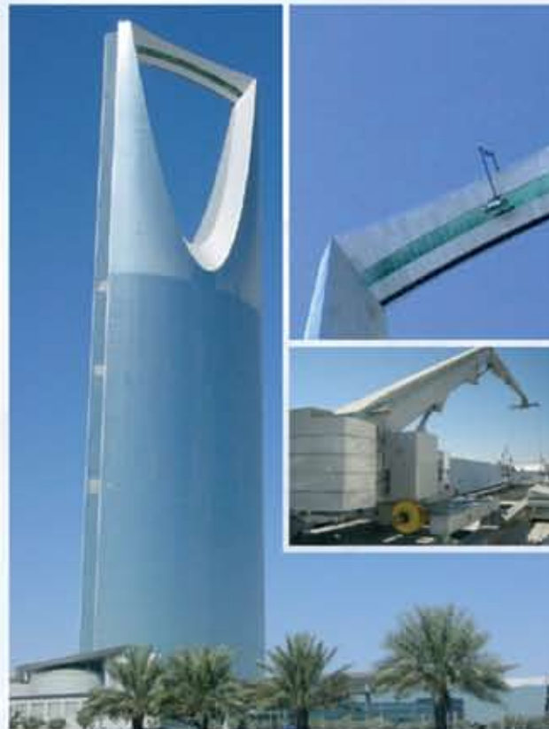
Type 6.1, track-based with vertical slewing articulated jib to reach recessed building areas
